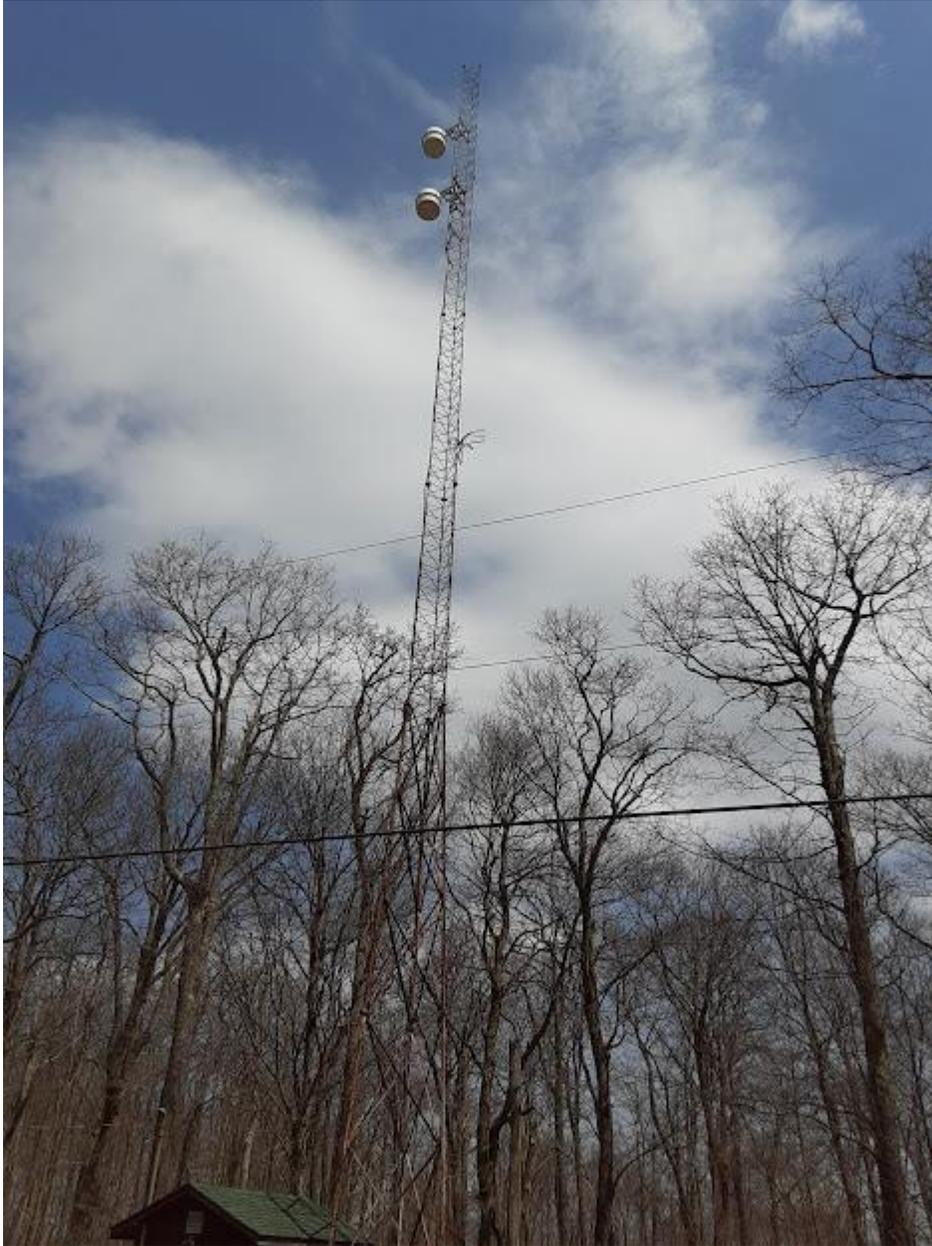
The photo above clearly shows the 2 bay antenna system installed at the site along with the STL link confirmed to match the azimuth between the site and the studio on Hunsrick Road.
