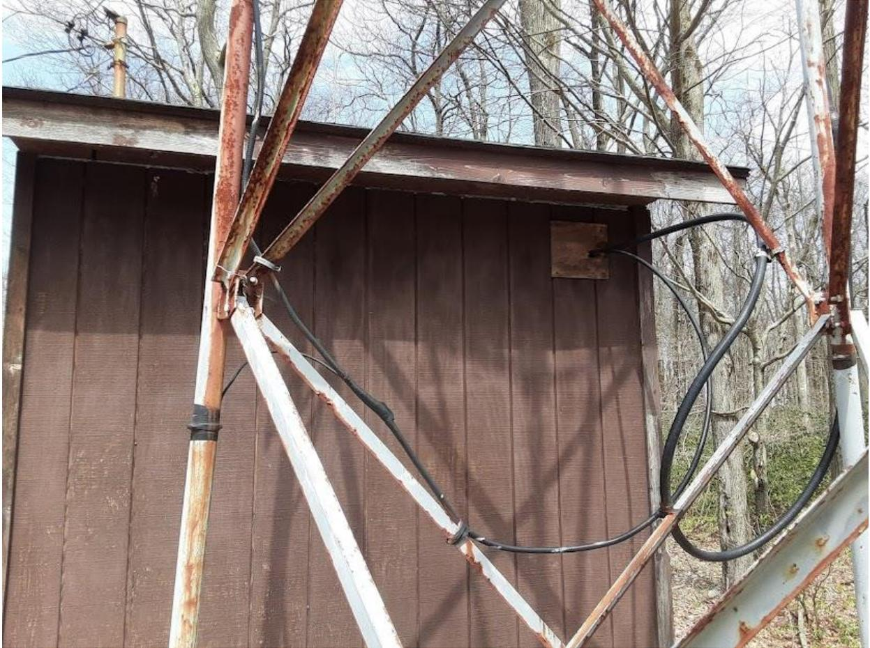
The photo above shows two lines between the shelter and tower, one going to the splitter for the 2 bay antennas and the other to the STL. This further validates that the second bay is not fed by a separate line, and is not an auxiliary or emergency antenna.
