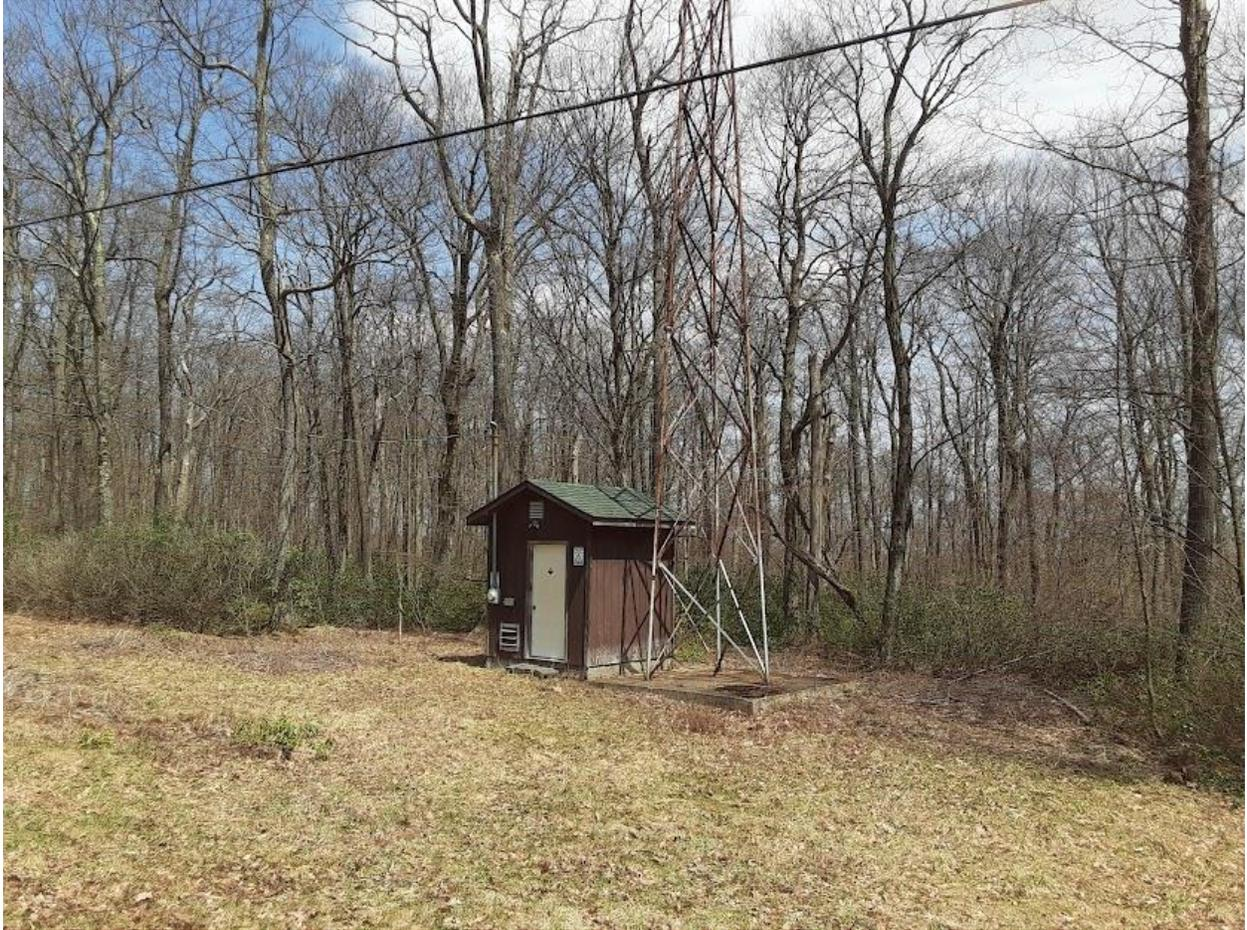
The photo above shows the WQZS equipment shelter and tower base. No fencing with warning sign exists at this facility as indicated on previous FCC application. In addition the building and site is not built in accordance with specifications indicated in lease paperwork submitted as part of an additional exhibit.
