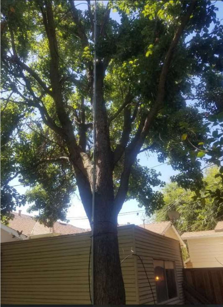
Coax running out of studio up tree mast to antenna
