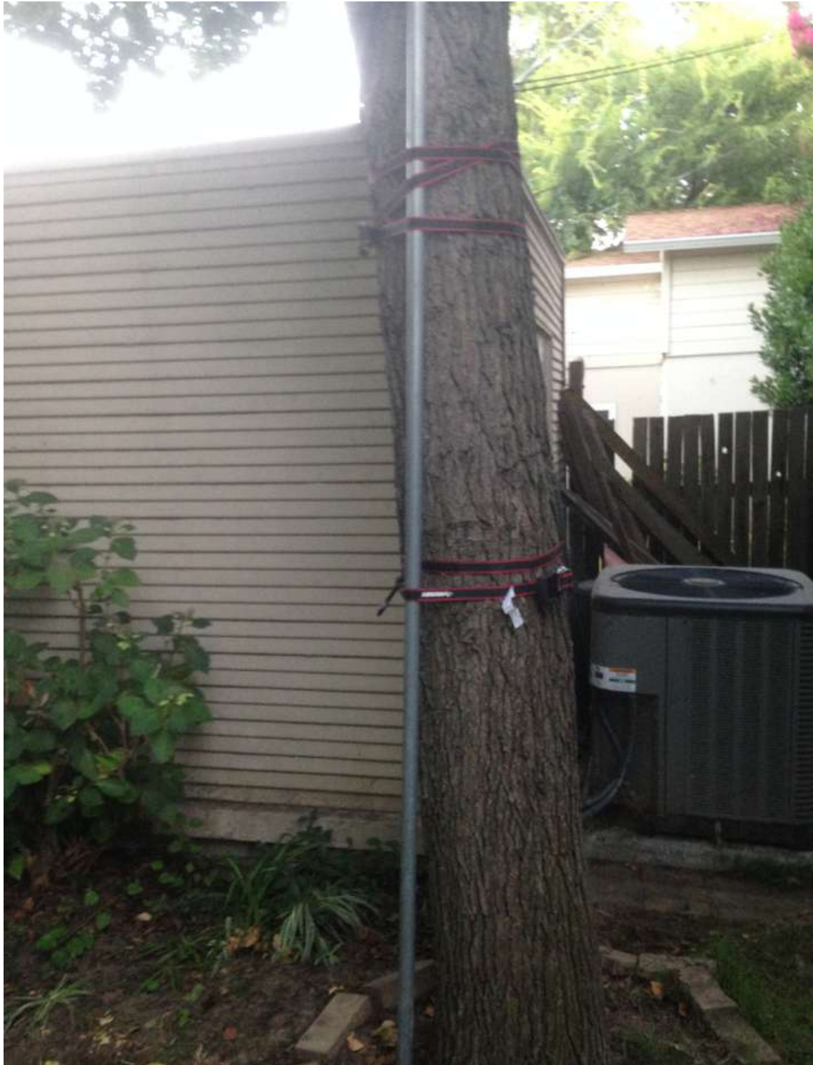
Bottom of mast, braced to tree and guyed above.
