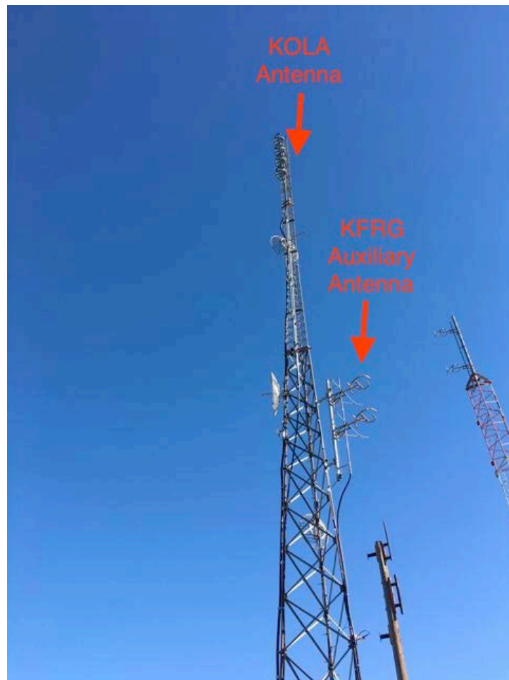
KOLA/KFRG Tower also showing KUCR tower near the center of radiation (COR) for KFRG and close to the COR for KOLA. No ground level REE issues were found.
