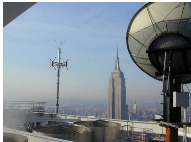
Figure 4. The FM backup antenna mounted near the southeast corner of the 4TS building. The Empire State Building is seen in the distance.
