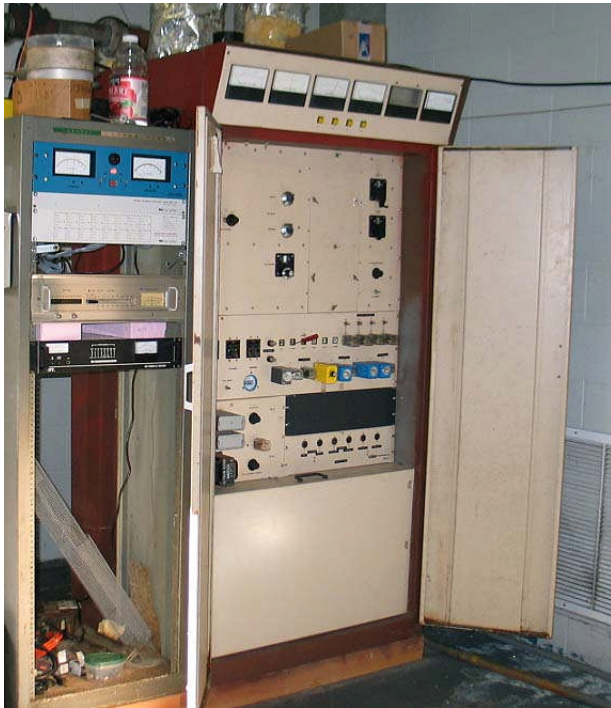
The KANO transmitter. A 1980 vintage CSI 20KW model.
