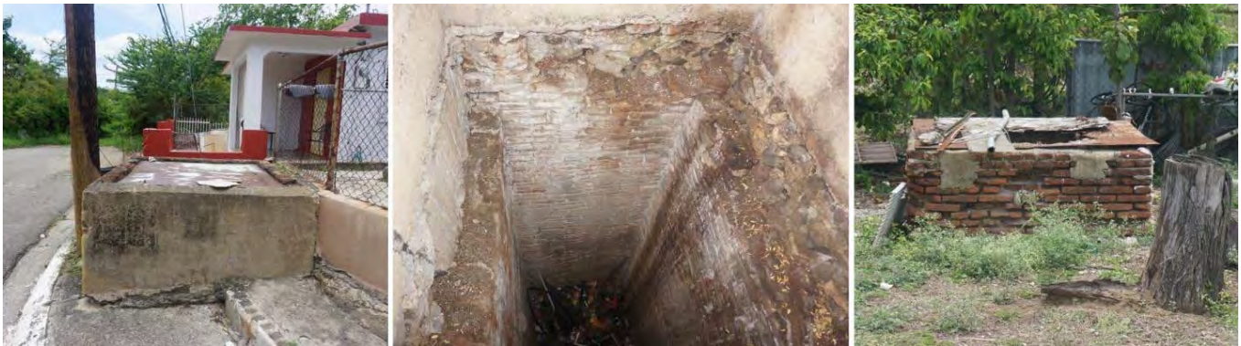
On the left, service manhole to the supply channel, located on a sidewalk of the El Ojo Community. In the center, detail of the service shaft inside a manhole. Right, manhole which features an advanced degree of damage by erosion, located in the backyard of a house.
