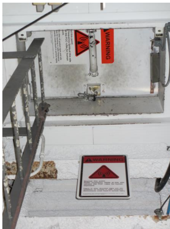
Photo 3: Interlocked Roof Access Hatch
