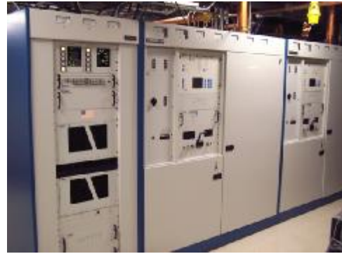
The two tube HPAs used by WRC-DT, Channel 48, have a combined output power level of 38.7 kW.
