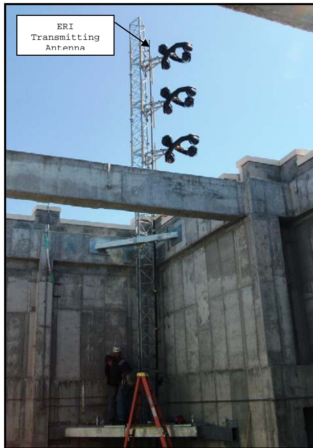
Photograph 1. Installed WCTZ(FM) Transmitting Antenna and Supporting Structure located on the upper rooftop level.
