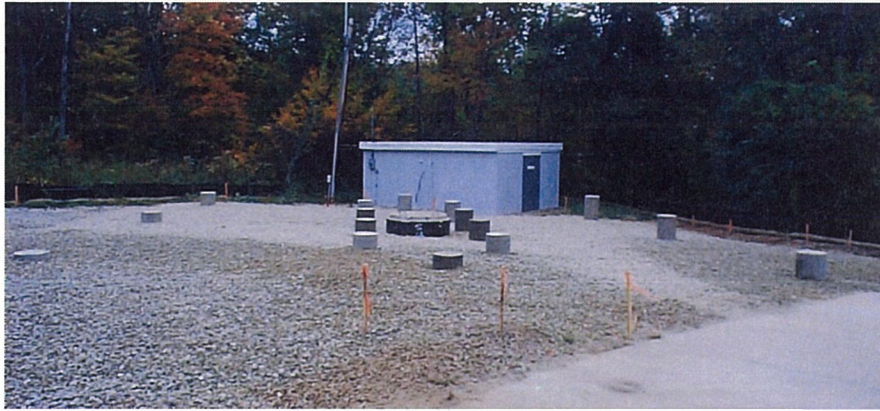
Platform Base Sonotubes Installed Near Transmitter Bldg.
