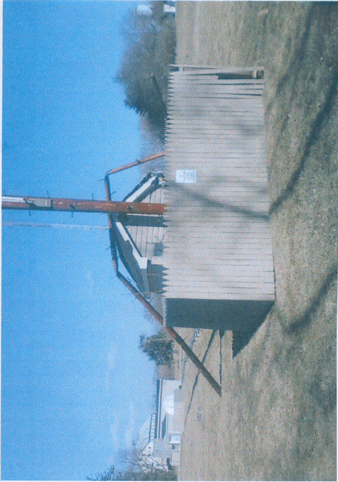
Fig. 1: Section of Collapsed WOYK Tower 3 Draped over ATU Building (NE view)
