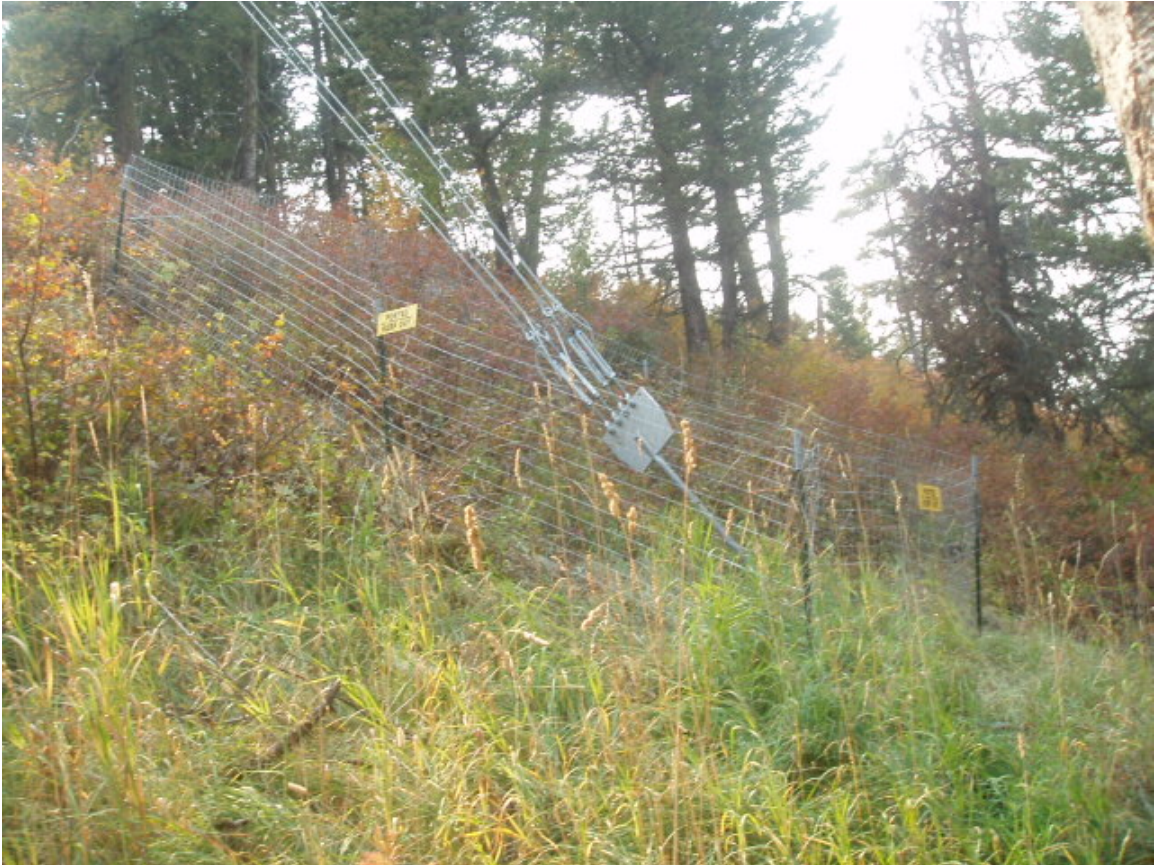
Fence surrounding Northern outer guy wires.
