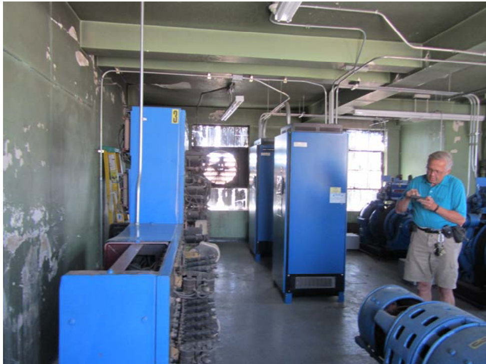
INTERIOR VIEW OF ELEVATOR CONTROL AND MOTOR ROOM
