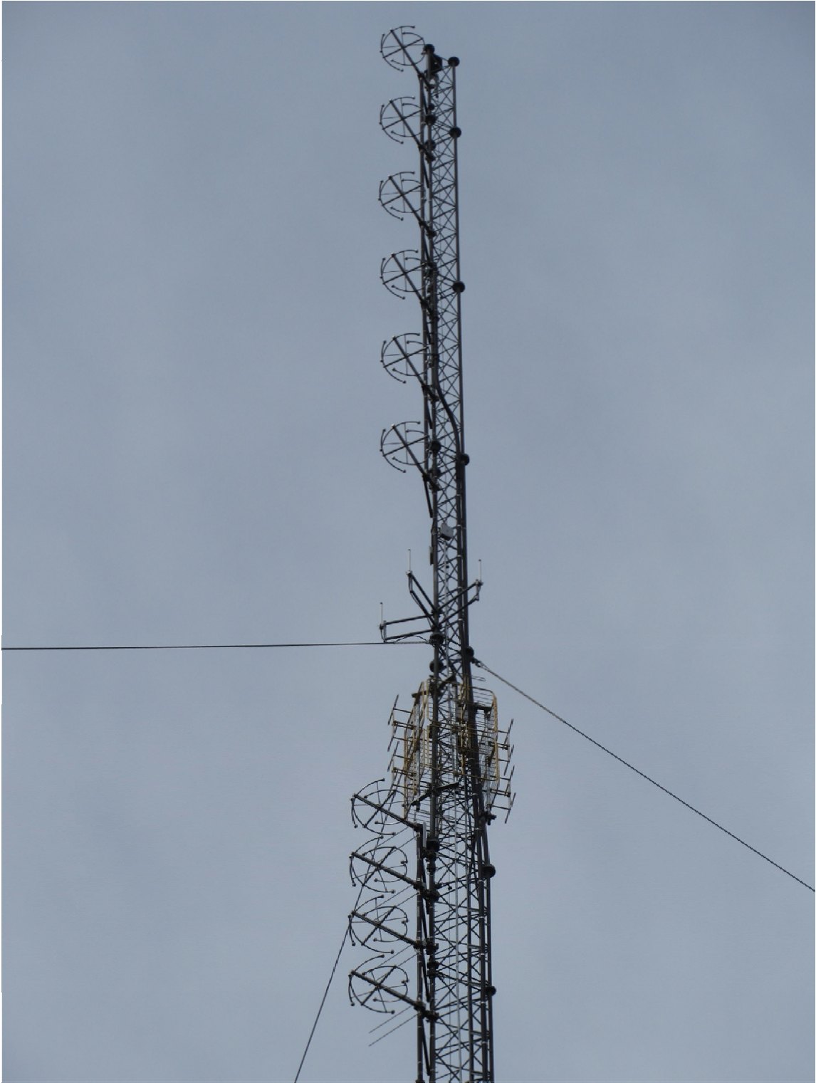
Close up view of the KTWS and KLRR common antenna at top of tower
