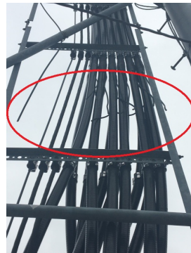
Visible cuts in Coax and cable grounds
