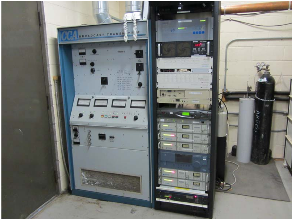
Inside view of transmitter building, KQAK transmitter and combiner
