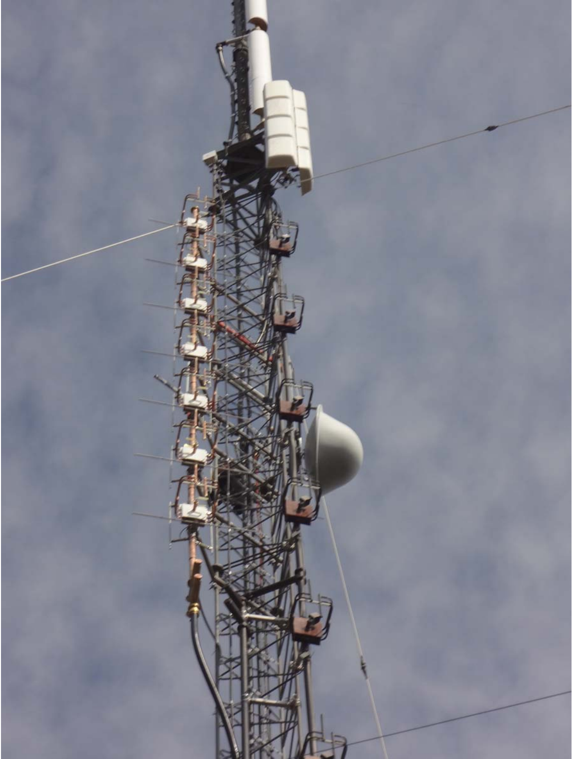
Close-up view of antennas. KLTW antenna is on left.
