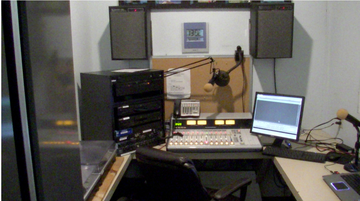
Studio 1 is the Production studio for training and pre-recording. Both studios feature professional broadcast consoles and audio playback gear. Community Producers master thier programs to a digital Audio Worstation running Adobe Audition editing software.
