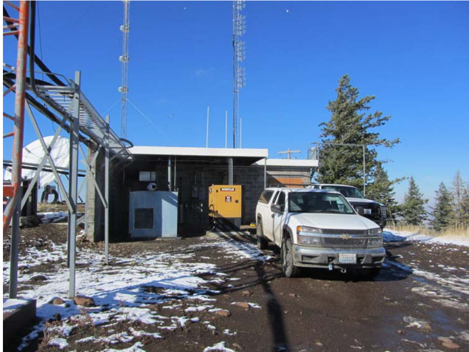
Parking area. Generators can be seen to the left of the pickup. Power company meters are behind the generators. Fuel tanks are located to the left of the building.
