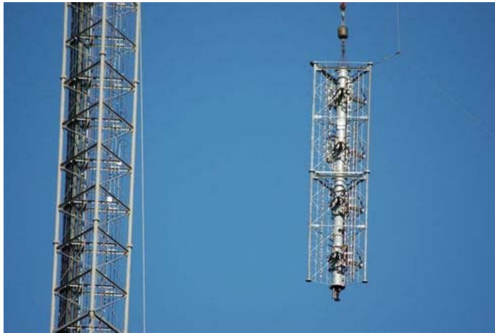
Senior Road Tower Group COGWHEEL Master FM Antenna installation of two sections in January 2006.
