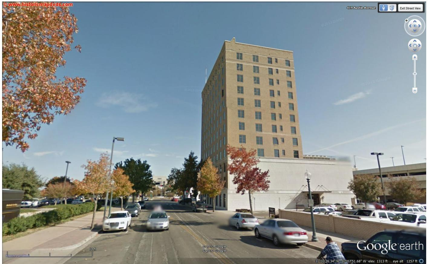
This building is a 12 story structure with standard 12 foot floor heights, plus the oversized height of the top floor of 18 feet. This brings the total building height to 150 feet above ground level. However, as previously stated, the interference zone lies at or above 173 feet above ground level, thus, this building is entirely below the interference zone, thus no population would be affected. The second building under consideration is depicted next.
