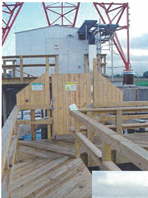
Left Center: The gate used to access Tower 2. There are stairs to the porch just beyond the gate. Each tower has a similar gate. All gates have appropriate RF safety signs. Tower 2 has the larger shelter to accommodate the phasor.
