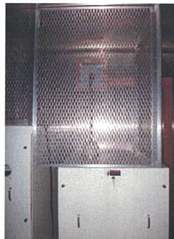
Below: All energized circuits are shielded to reduce RF field levels to a minimum and to prevent inadvertent contact.
