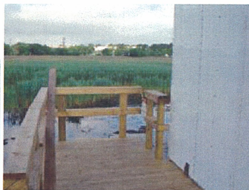
Above: Tower 2 porch looking westward. Access to the tower leg with the feed line is made from this point. An additional chain and RF hazard sign is about to be added to restrict access to this end of the porch.
