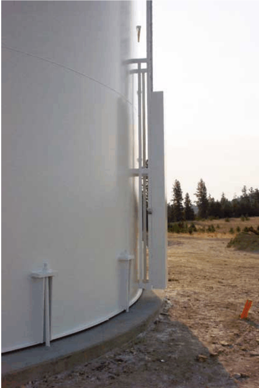
Photo of the locked panel preventing unauthorized persons from accessing the climbing ladder on the water tower.
