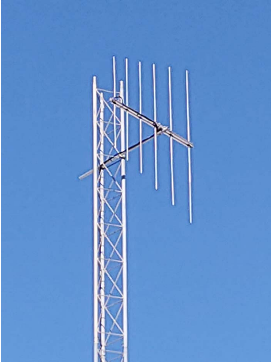
NCG Comet CD-95Y antenna shown installed on existing tower. (Photo taken 01/07/2021)
