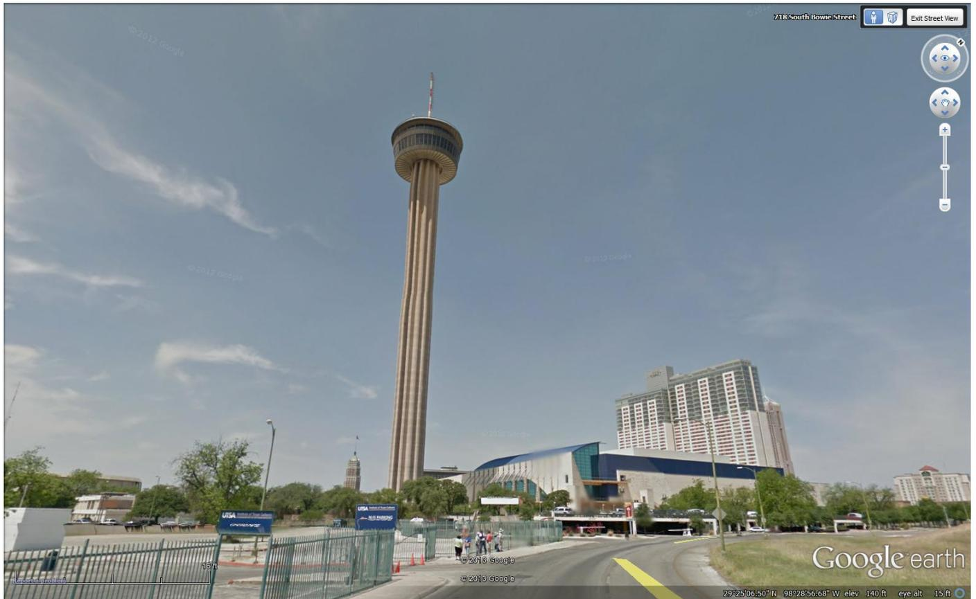
The proposed antenna would be roof mounted on the platform on the Tower of the Americas depicted in the photograph. The closest structure to the Tower of any substantial height is the Hyatt hotel, depicted to the right of the Tower in the photograph. The closest point of the Hyatt is at least 250 meters from the Tower, and as such would be unaffected by the potential interference region.
