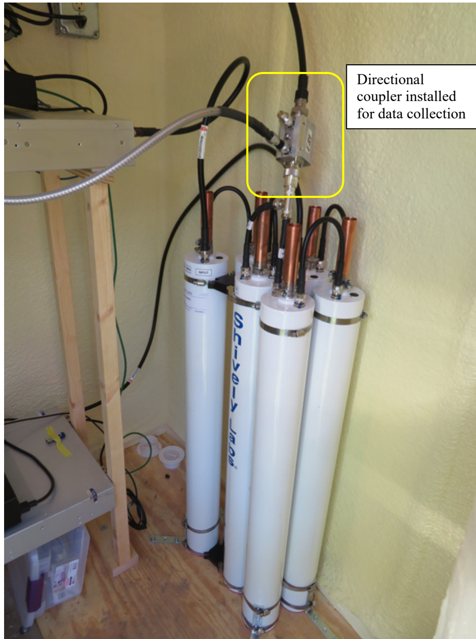
Figure 2 – Photo of Shively Branch Combiner with Directional Coupler Installed
