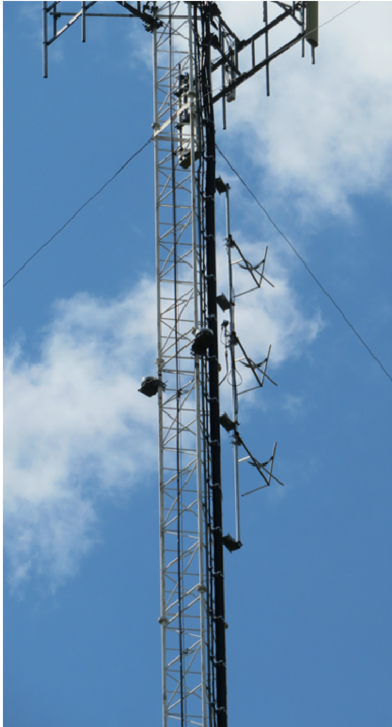
Figure 1 – Photo of Shively 6832-3 (3-Bay) Antenna, As Installed
