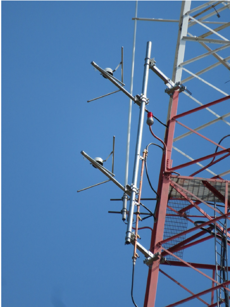
Figure 1 – Photo of Shively 6842-2P (2-Bay) Antenna, As Installed
