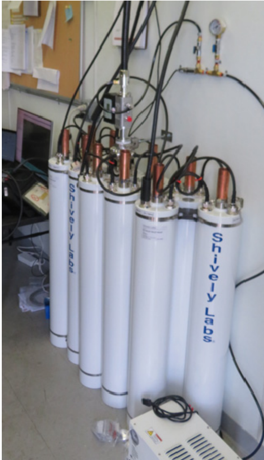
Figure 2 – Photo of Shively Branch Combiner and Directional Coupler
