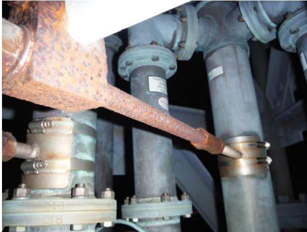
Figure 5 – Rusty Bolt Syndrome Is a Well-Known PIM Cause (Found on SBA Tower)
