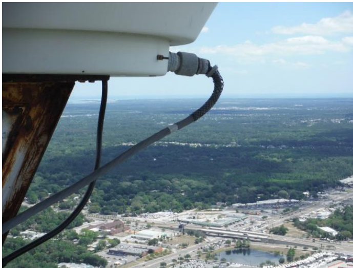
Figure 7 – Loose Connectors & Connectors with Broken Cable Connections, as Found at SBA Tower, Can Contribute to PIM Generation
