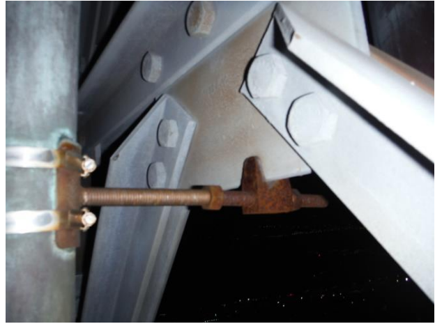
Figure 6 – Rusty Bolt Example Found in Transmission Line Support on SBA Tower
