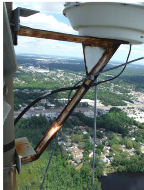
Figure 8 – Rusty Mounting Hardware Can Lead to PIM as in This Mount on the SBA Tower
