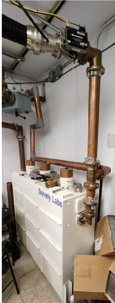
Figure 2 – Configuration of Combiner Tee
