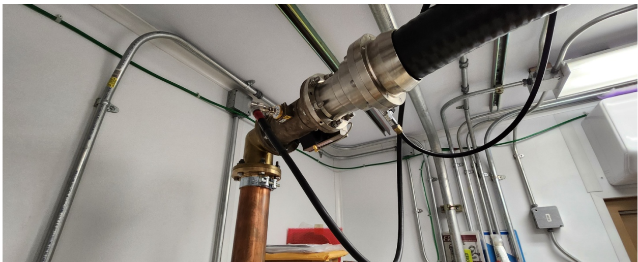
Figure 3 – Directional Coupler at Output of Combiner System
