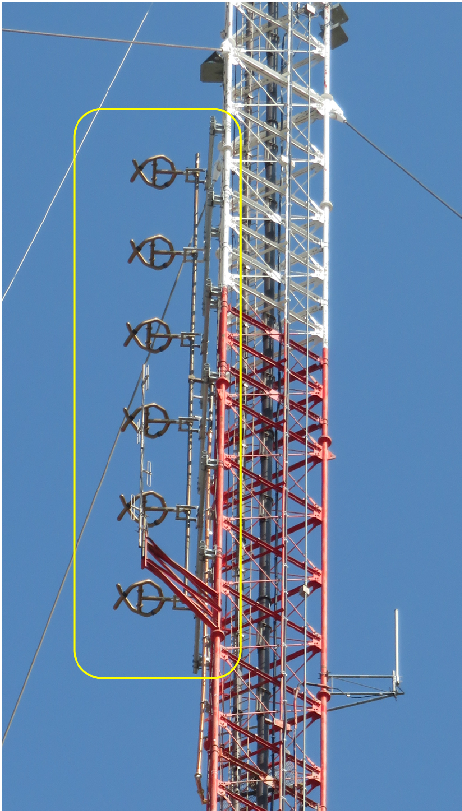
Figure 4 – Combined System Antenna, ERI Model SHPX-6AC-SP
