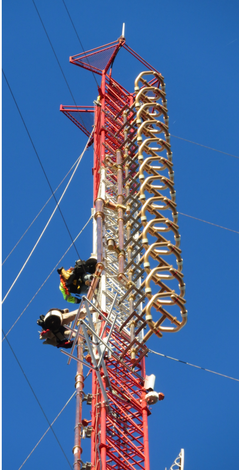
Figure 3 – Combined System Antenna, ERI Model SHPB-12C6-SP
