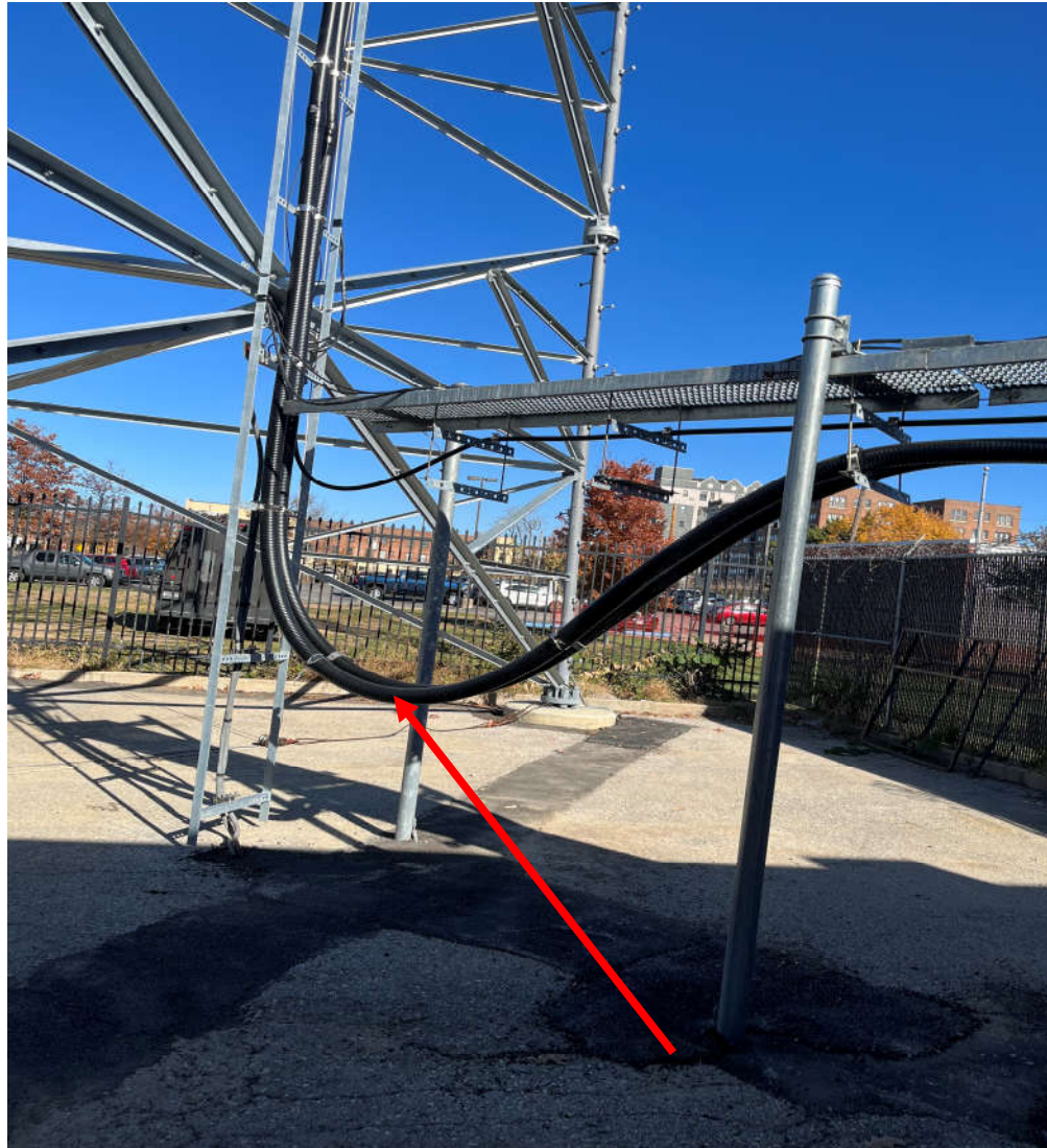
Photo 3: Drip Loop at Tower Base for 95.5 and 104.1 MHz. Antennas.
