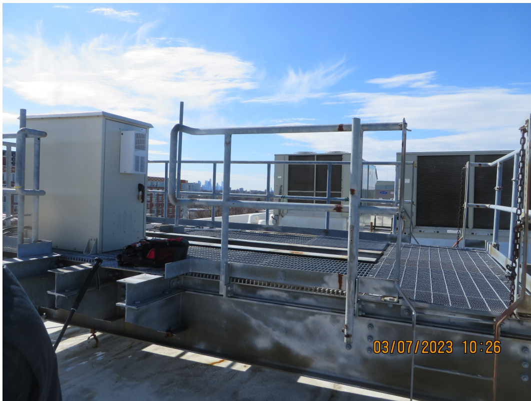
Gridwork platform with the transmitter cabinet
