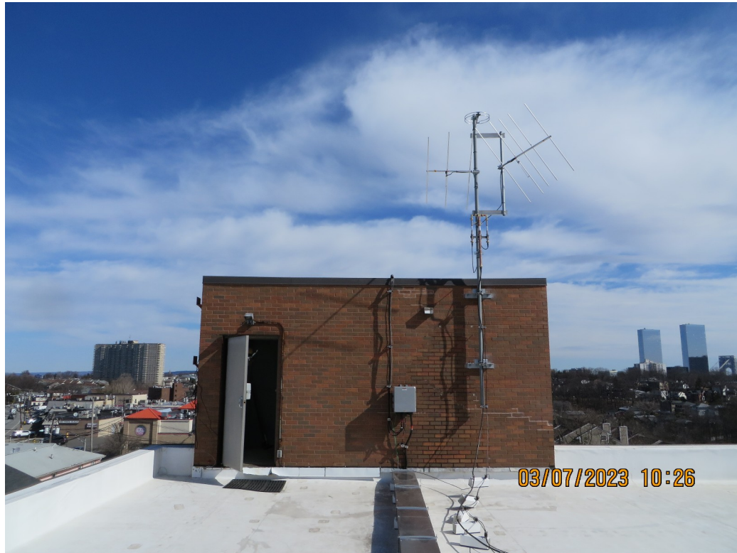
Antenna mounted on the penthouse wall
