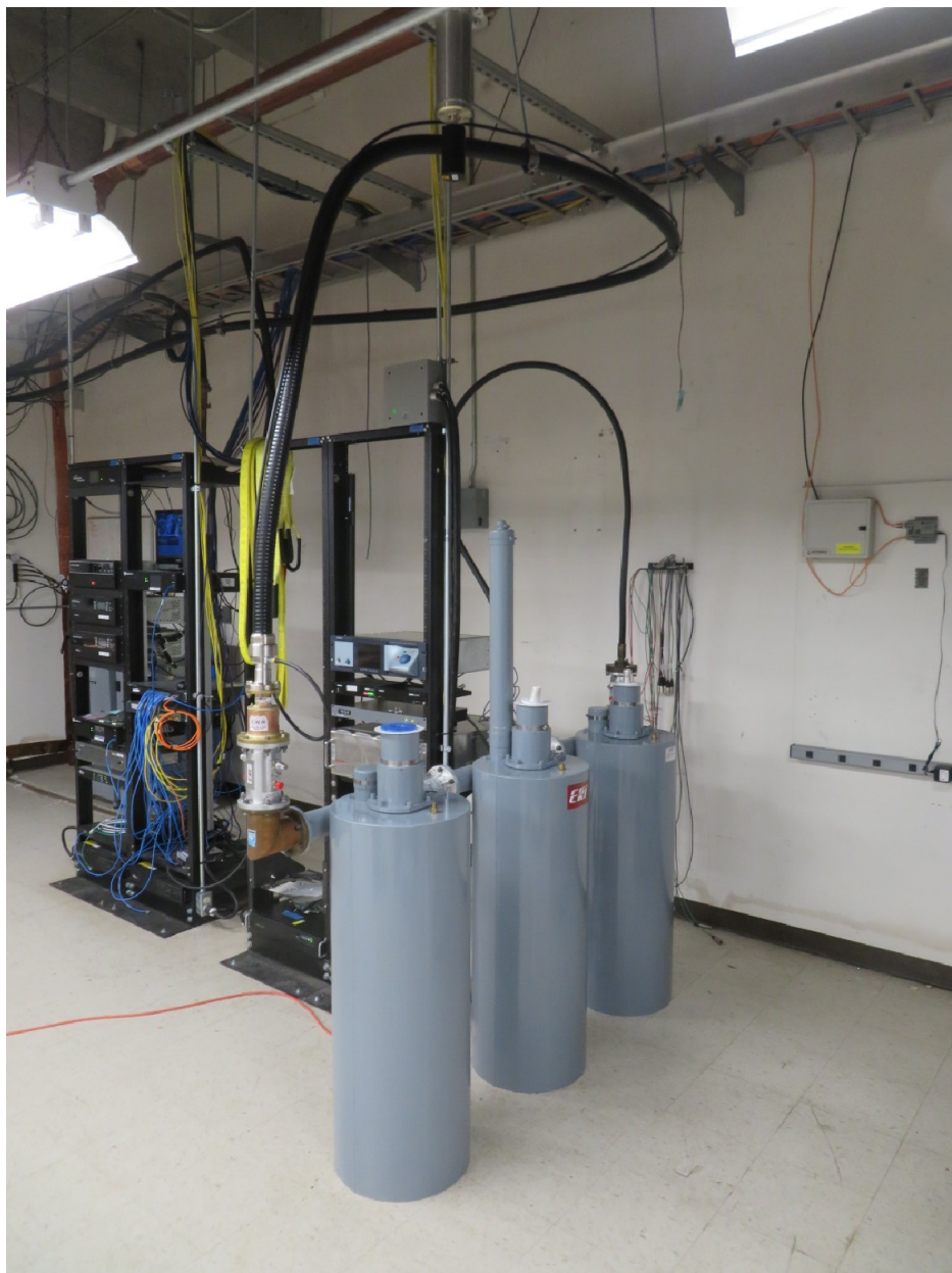
Figure 2 – Photo of ERI Notch Filter
