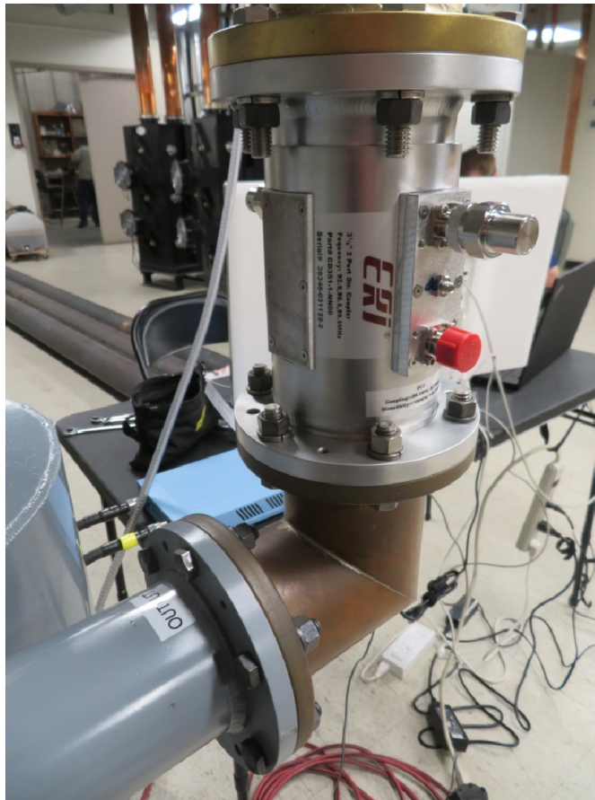
Figure 3 – Directional Coupler at Output of Combiner System
