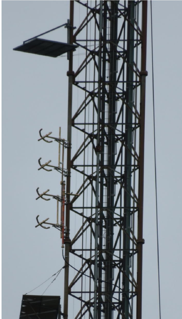
Figure 1 – Photo of ERI Axiom SHPXA-4BC-HW-SP Antenna and Ice Shield
