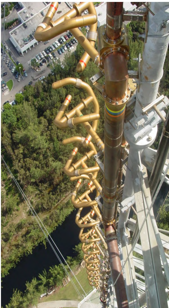
AXIOM™ SHPXA-16BC-HW-SP Broad Band FM Antenna owned by American Tower in Miami, Florida
