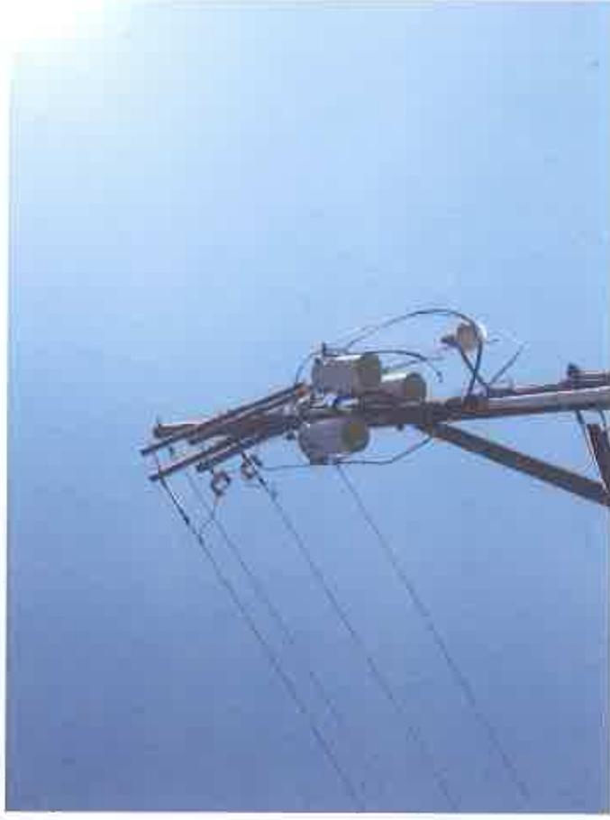
Pole mounted electrical transformers on project site labeled as being "Non PCB" containing
