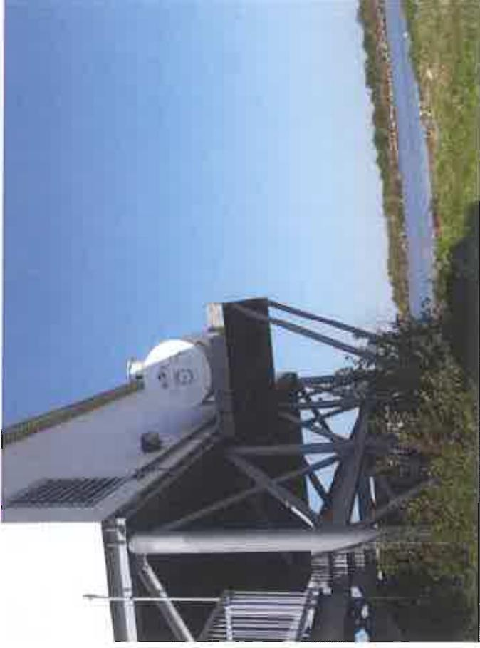
One approximately 500 gallon capacity above ground storage tank for emergency generator fuel for raised equipment building
