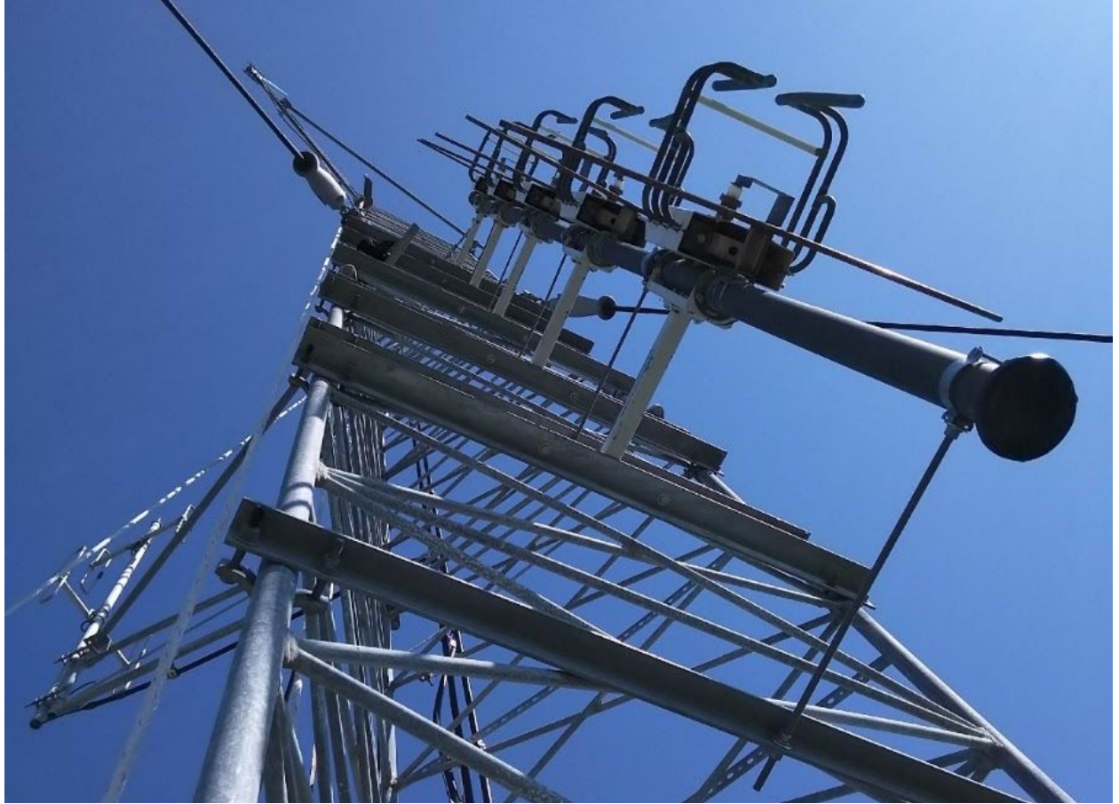
Monday August 3rd, 2020 - Antenna Mounted back on the tower with custom machined mounts.
