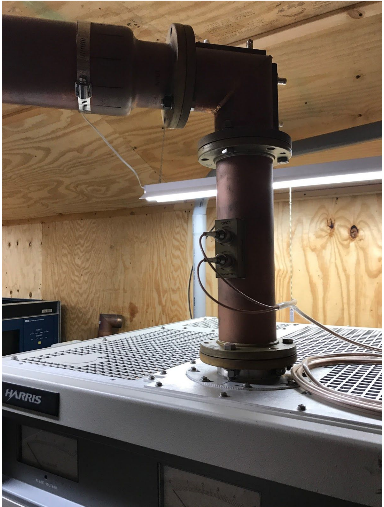
Friday August 7th - Hardline going into the new Transmitter.
