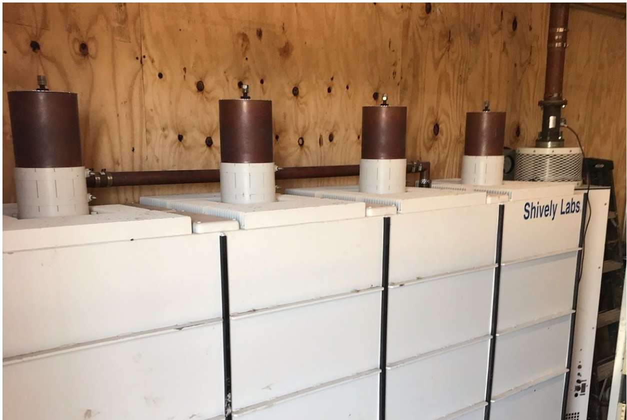
Monday August 3rd - Picture of the filter on one wall of the transmitter building.
