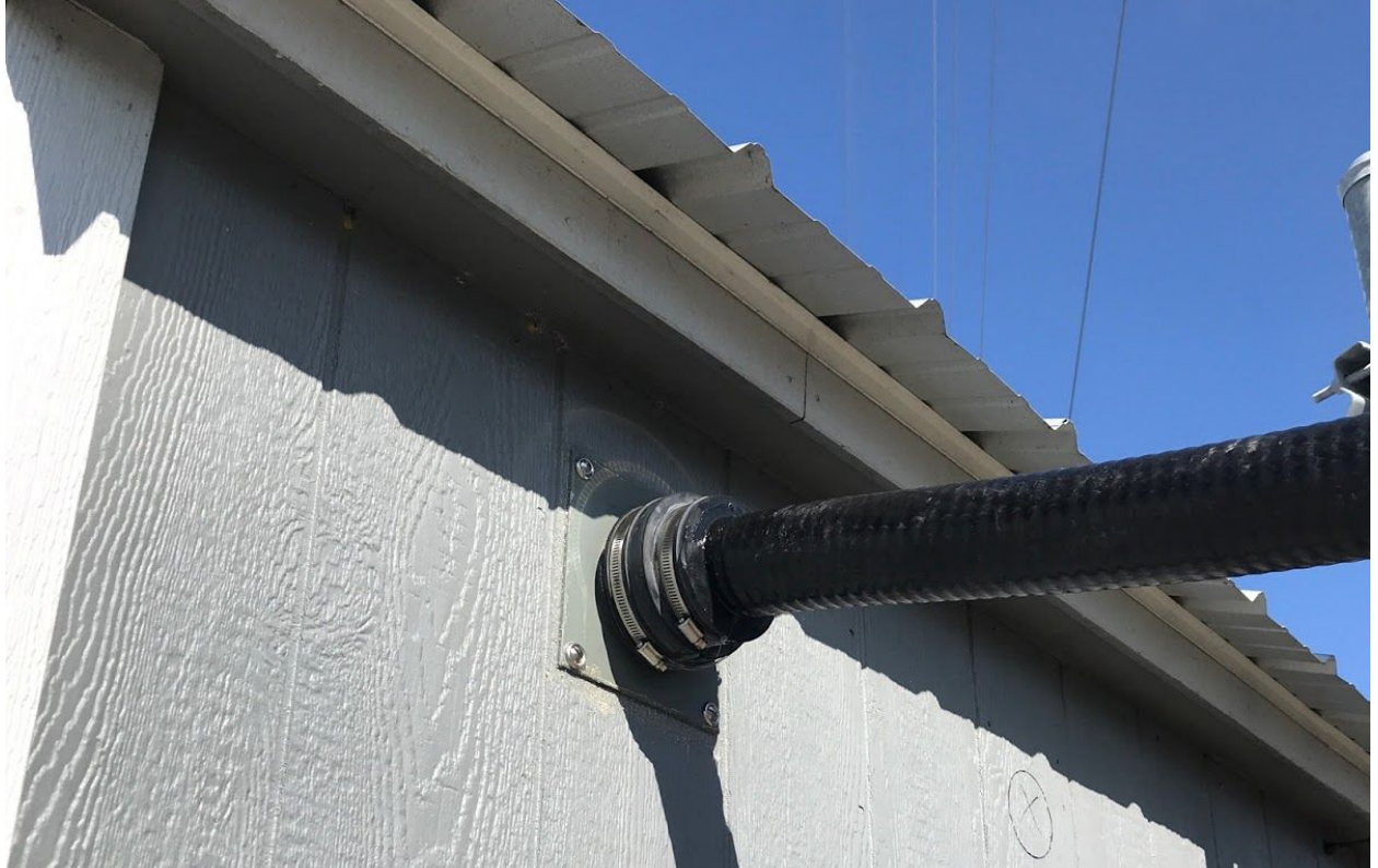
Friday August 7th, 2020 - Hardline into the building from the antenna.
