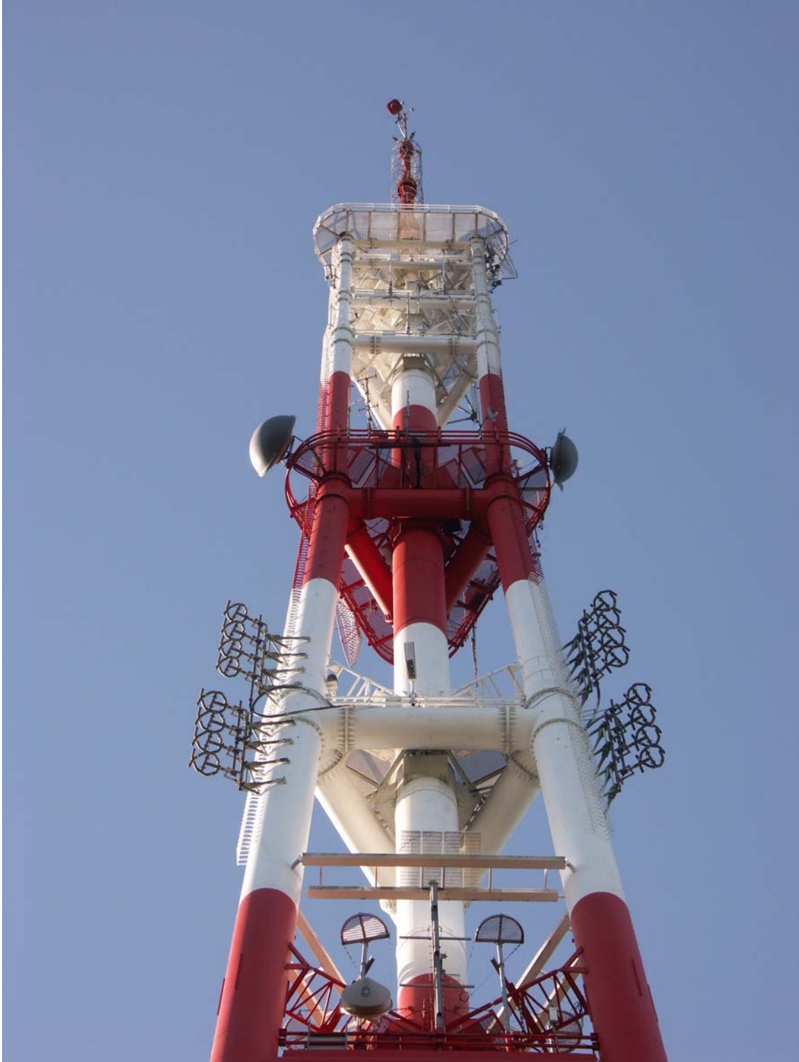
Close-up view of tower structure. Antenna with radome at very top is KNRK. Spiral antenna below it is combined antenna for all other stations. Auxiliary antennas can be seen on legs of structure.
