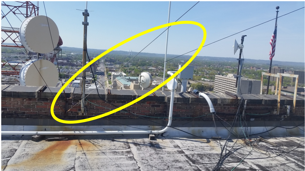
Figure 9 - Typical Guy Anchoring at Roof Level for WFMP-LP Tower on Upper Roof
