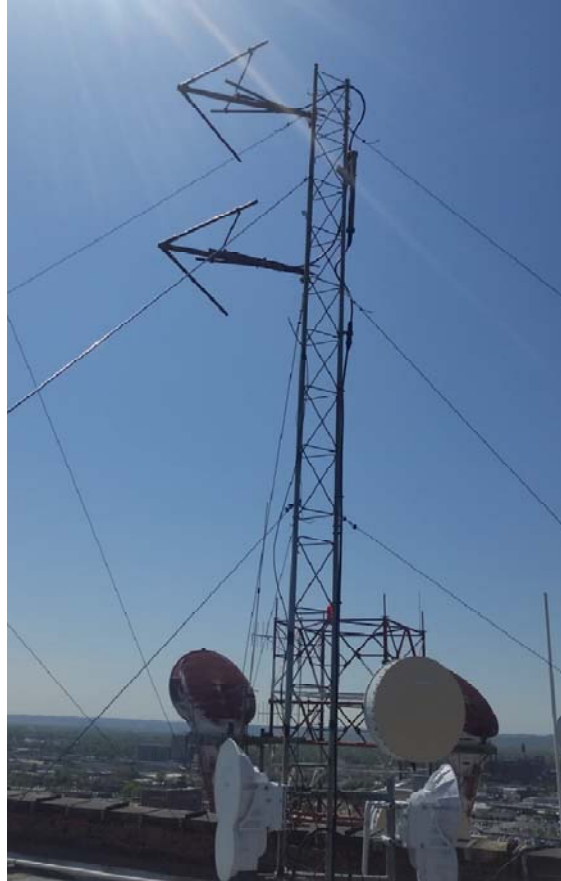
Figure 8 - Guyed WFMP-LP Tower on Upper Roof
