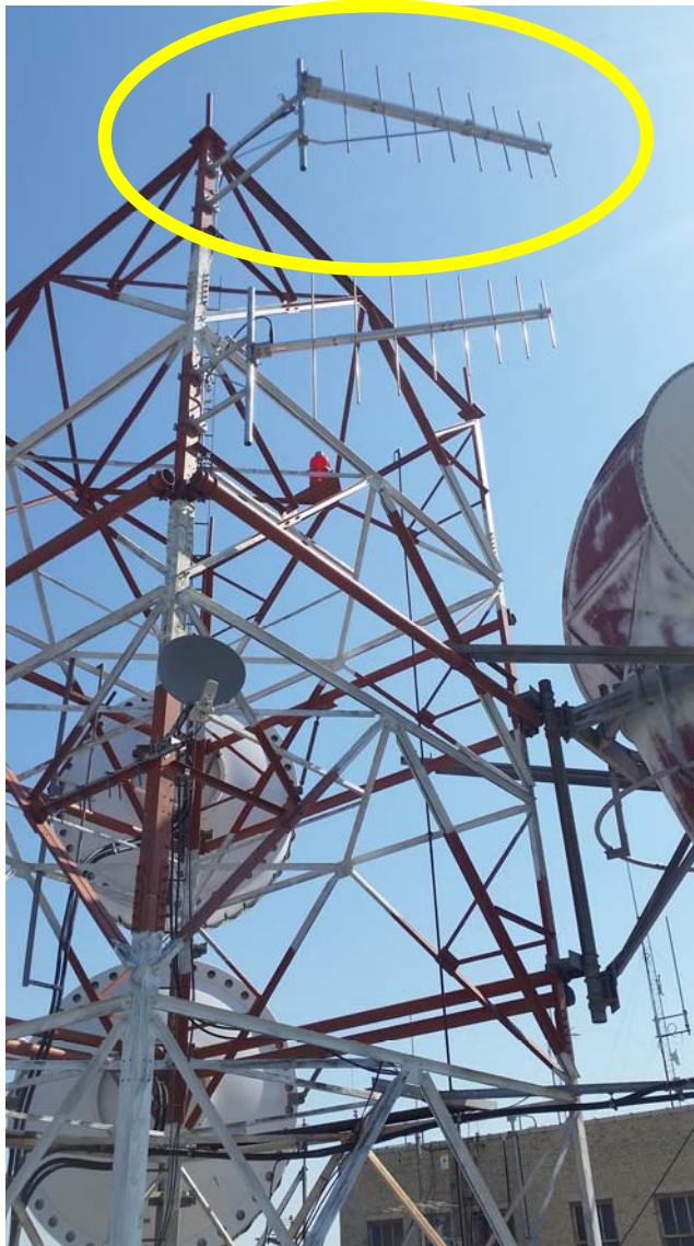
Figure 3 - W250BD Antenna (Top Bay Transmits)
