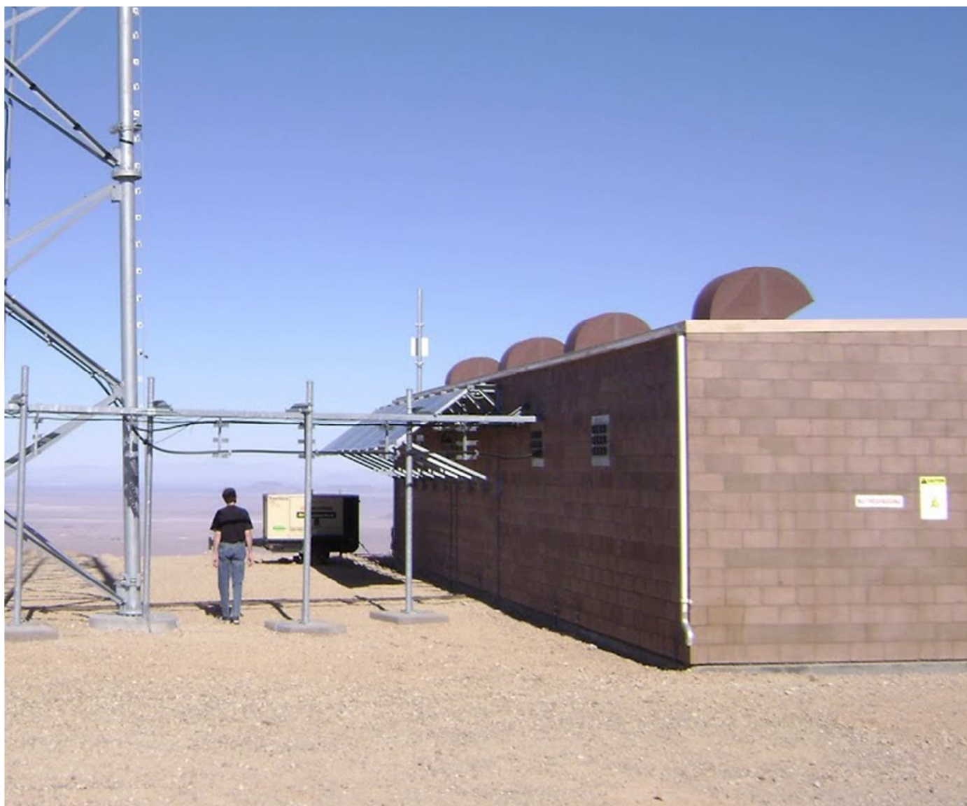
Tower base has no climbing spikes at ground level.
